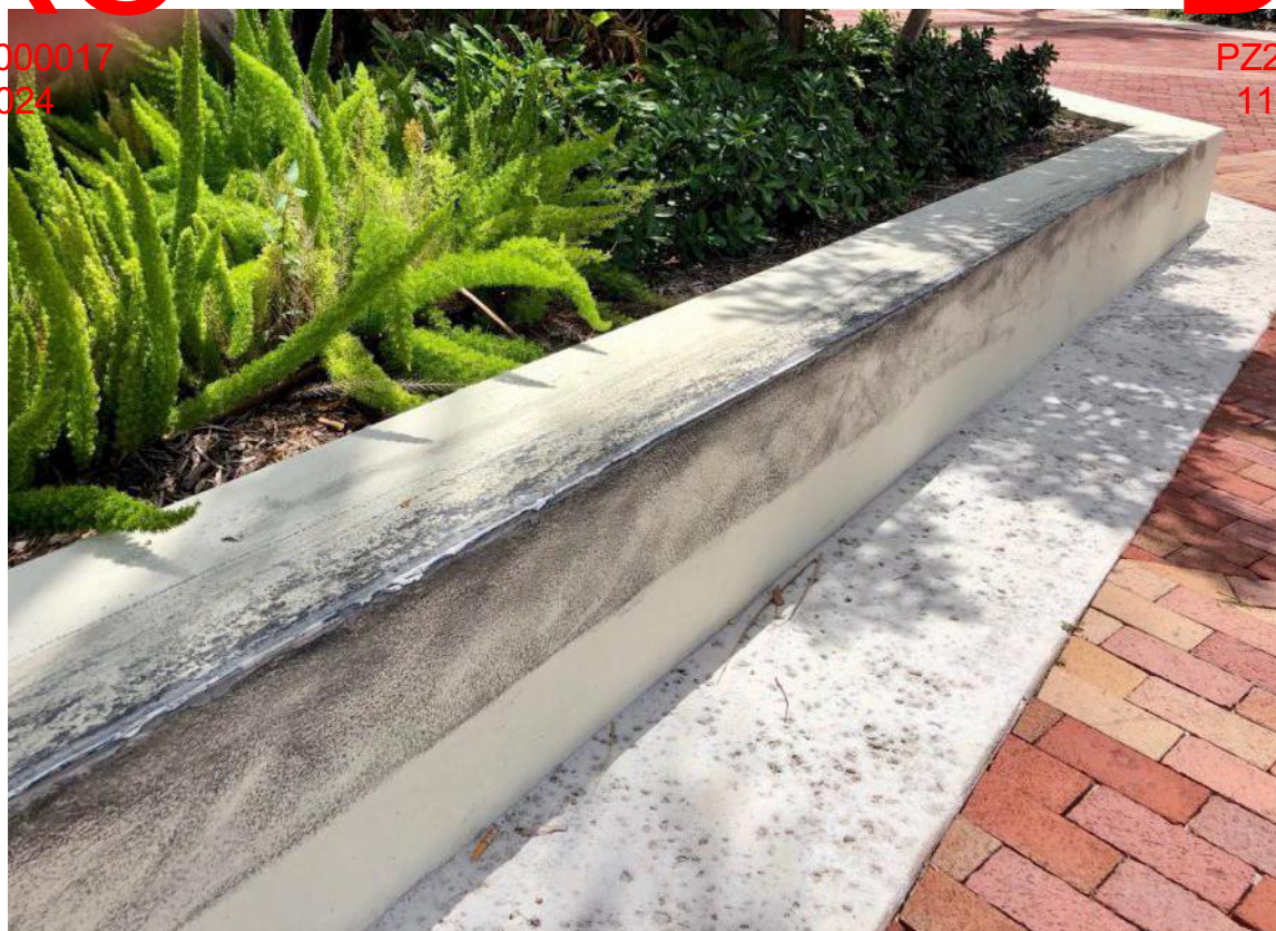
An example of damage from skateboarders to an unprotected retaining wall surface.
