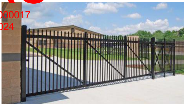
Examples of sliding vehicle gates.
