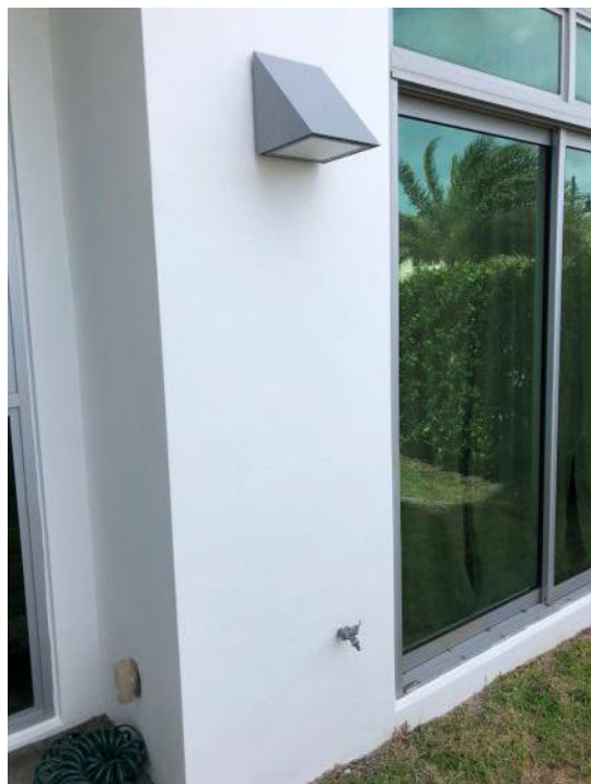
Examples of low maintenance shielded LED lighting
