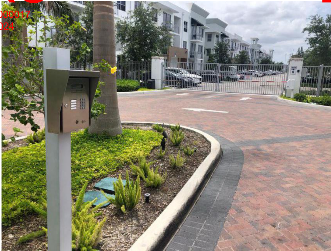
An example of a gate entry system, intercom, and turn around lane.
