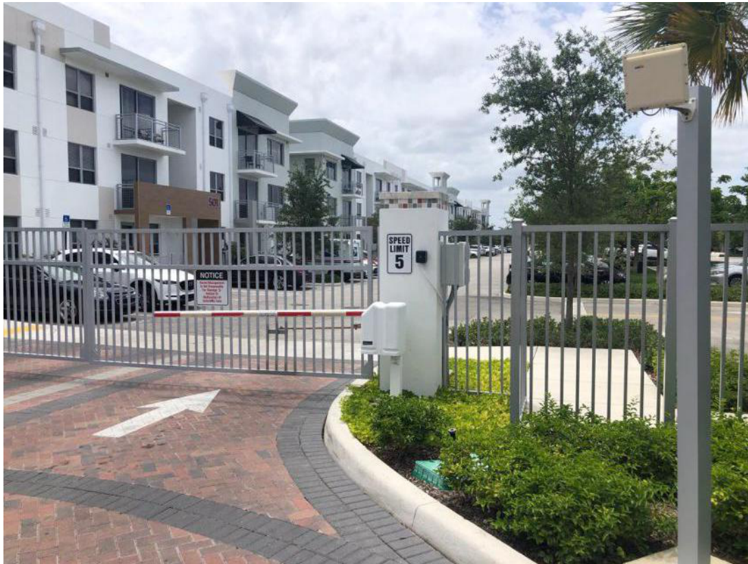
The reader on the right picks up the signals from decals or RFID stickers placed on residents' cars. The gate arm goes down after the car enters to stop tailgating.
