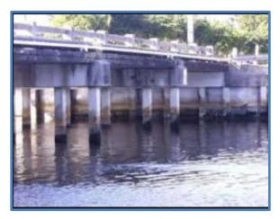
• McNab Bridge Renovation: This structure is 150' long, 5 span, 4 lanes with sidewalks on each side. Type II AASHTO girder bridge with a continuous cast in place and prestressed concrete pile foundation. Lakdas services as the Project Engineer and was responsible for the overall design of the bridge and performed Construction Engineering Inspections (CEI) services with supporting inspection staff.
