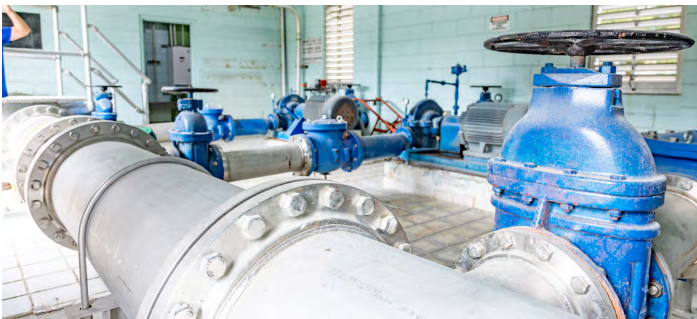
► City of Palm Coast - Pump Header Replacement
