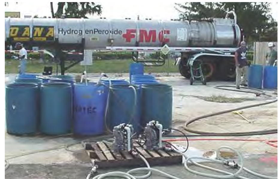
Former Hanner's Cleaners Chemical Oxidation Injections
