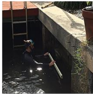
Stormwater outfall assessment.
