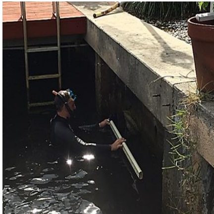
Stormwater outfall assessment.
