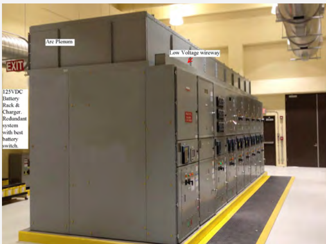
Example of a 5-kV switchgear design, which will replace the existing obsolete main switchgear in the Pumps 5-6 building.
