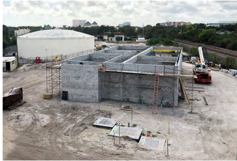
New Pump Station Construction at District 1B1.
