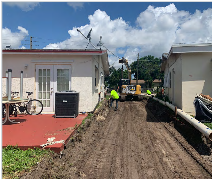
Baxter & Woodman provided CEI Services for Pompano Beach's Esquire Lakes project.
