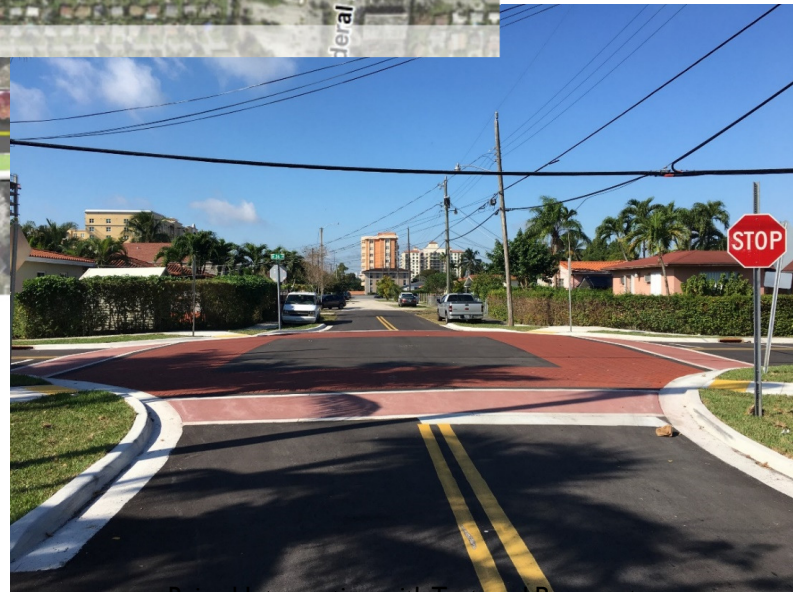
Raised Intersection with Textured Pavement
