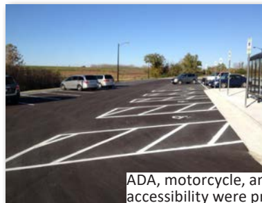
New lighting was included in the project. The perimeter of the lot was curbed and guttered to control storm water.
