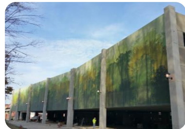
GARAGE SCREENING EXAMPLES
