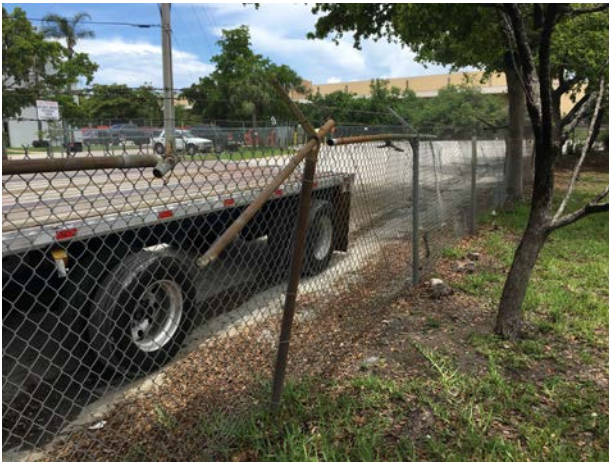
The North boundary is presently the primary access and egress points to the plant on NW 18 th Street. There are two gates openings. Both gates are left open and have been damaged and non-operational. The barbed wire on the top of the chain link fencing has been damaged and not consistent.
