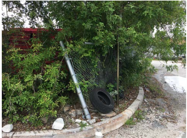
The North boundary is presently the primary access and egress points to the plant on NW 18 th Street. There are two gates openings. Both gates are left open and have been damaged and non-operational. The barbed wire on the top of the chain link fencing has been damaged and not consistent.
