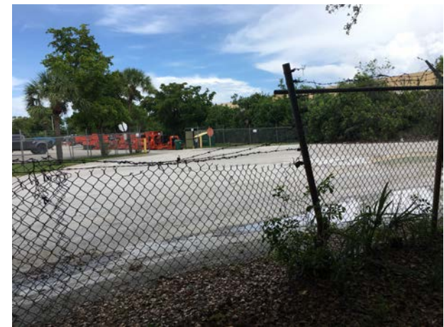
The North boundary is presently the primary access and egress points to the plant on NW 18 th Street. There are two gates openings. Both gates are left open and have been damaged and non-operational. The barbed wire on the top of the chain link fencing has been damaged and not consistent.
