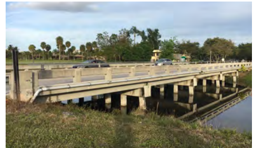
North Palm Aire Bridge
