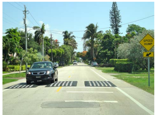
Examples of well-placed and marked speed humps for speed control. The parking lots is under natural surveillance from the windows of the adjacent apartment building unit.
