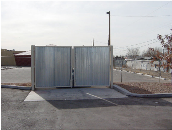
Additional examples of good CPTED design dumpsters, with good shielding, raised gates off the floor, lockable gates, and difficult to climb and sit on walls.
