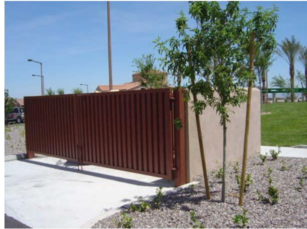
Additional examples of good CPTED design dumpsters, with good shielding, raised gates off the floor, lockable gates, and difficult to climb and sit on walls.
