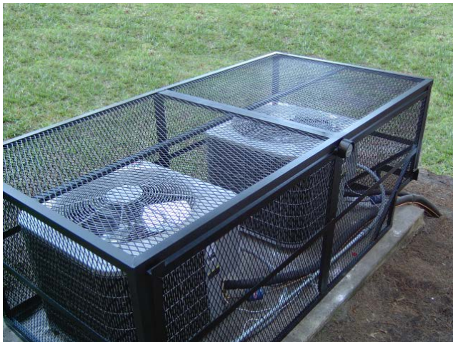
Examples of protecting the AC compressors on ground level.
