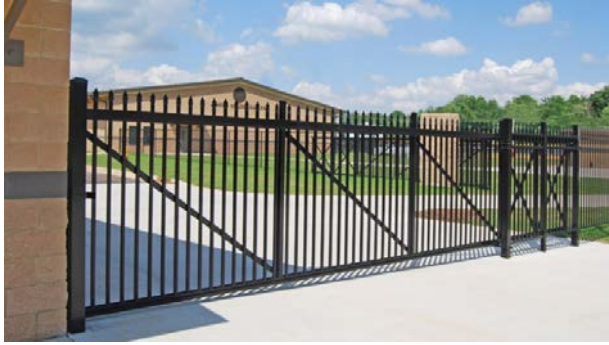
Examples of sliding vehicle gates.
