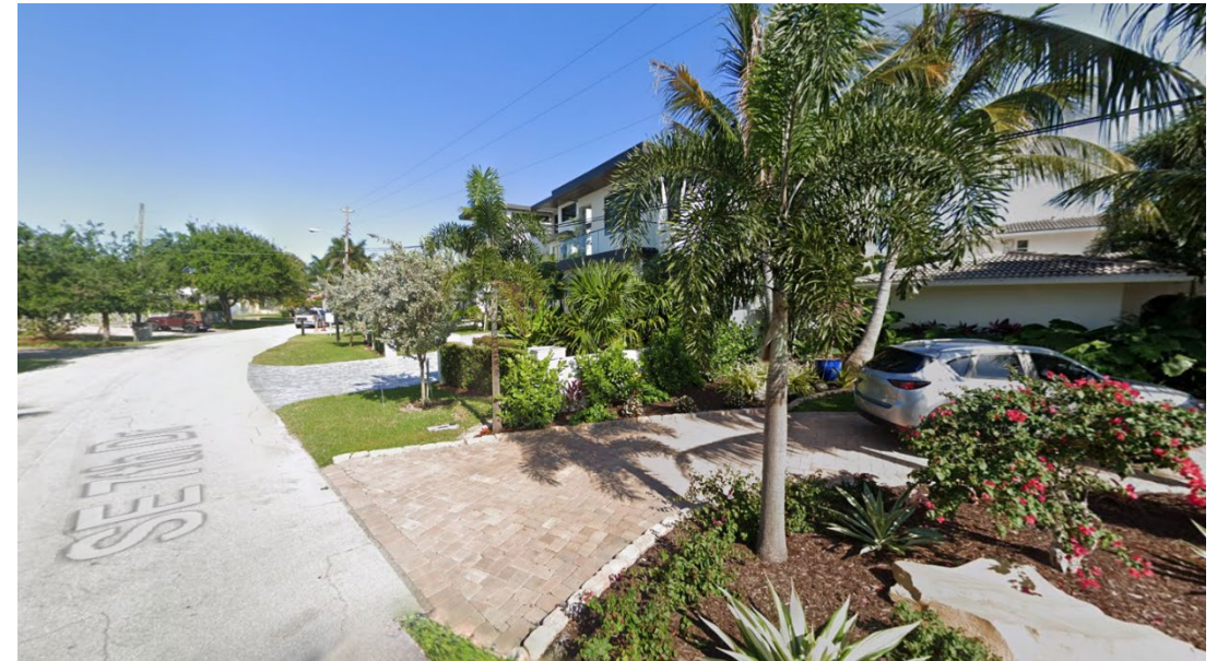
View of retaining wall with landscaping
