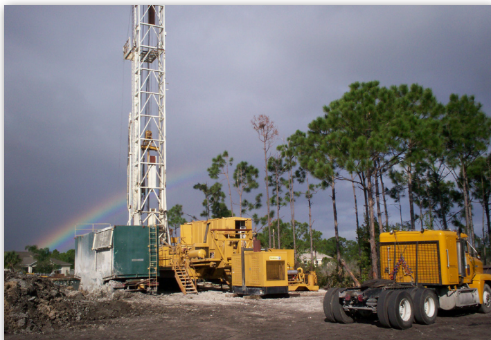
Port St. Lucie Well Construction
