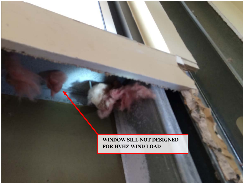
Photo 11: Filter Gallery Expansion - Window Sill Framing
