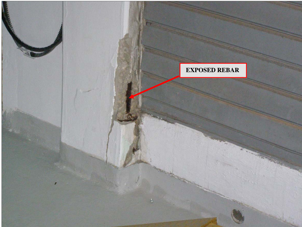
Photo 19: Column Damage in Generator Room
