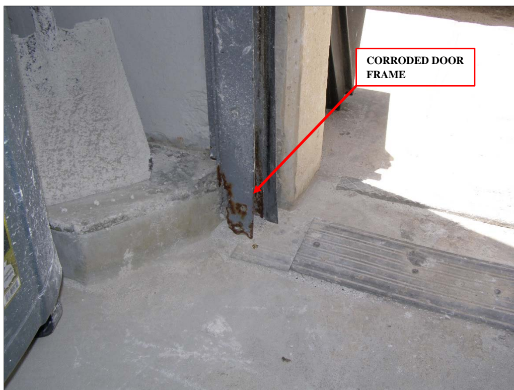
Photo 27: Overhead Door Frame Corrosion
