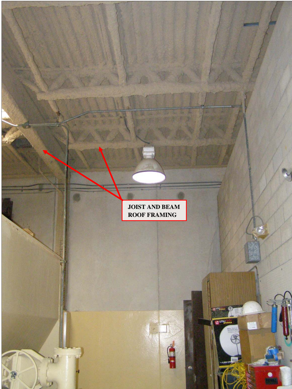
Photo 30: Typical Roof Framing
