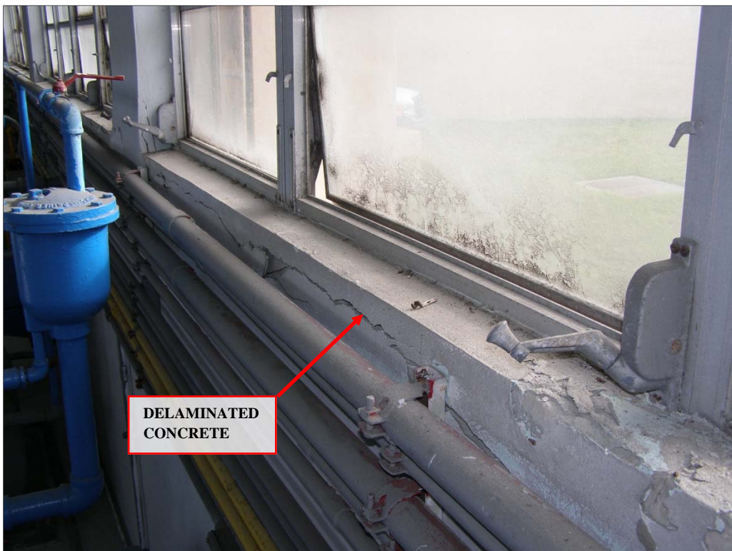
Photo 18: Window Sill Deterioration in Pump Room
