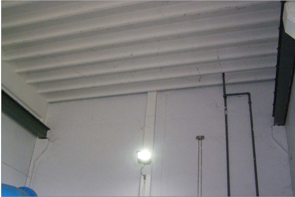
Photo 3: Typical Double Tee Roof Structure
