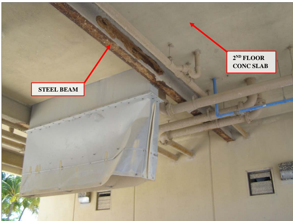
Photo 29: 2 nd Floor Framing Corrosion
