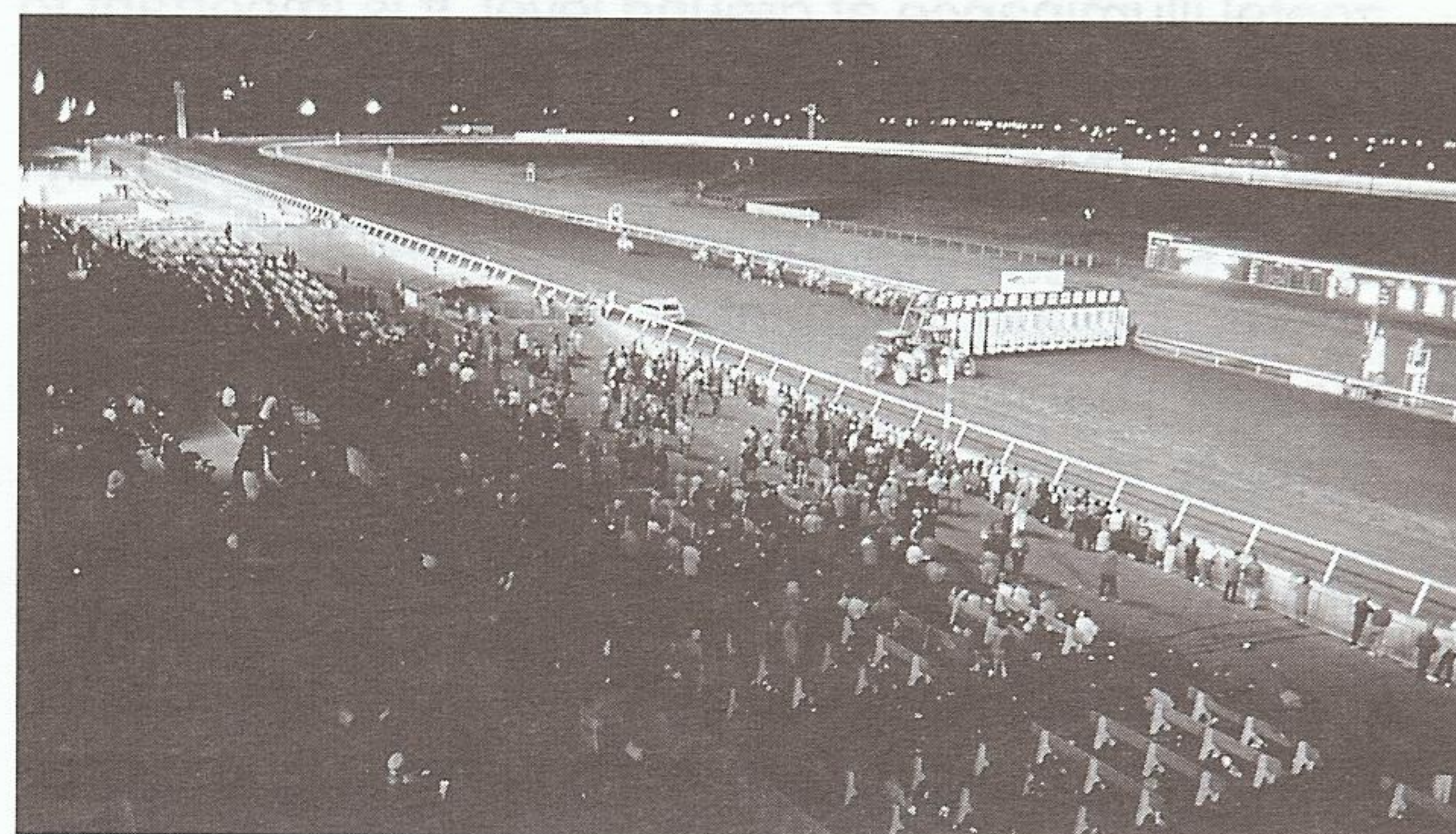
Figure 1. This racetrack is lighted by clustered banks on individual structural towers to provide the lighting needs of both contestants and a large number of spectators.
