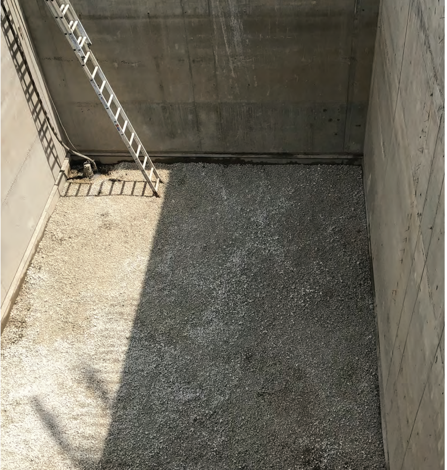
HARD ROCK STORM WATER STATION PRIOR TO INTERIOR CONCRETE WORK
