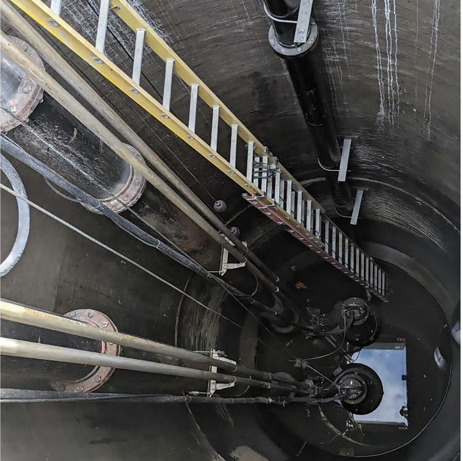
TYPICAL LIFT STATION PIPING IN PROGRESS IN WEST PALM BEACH
