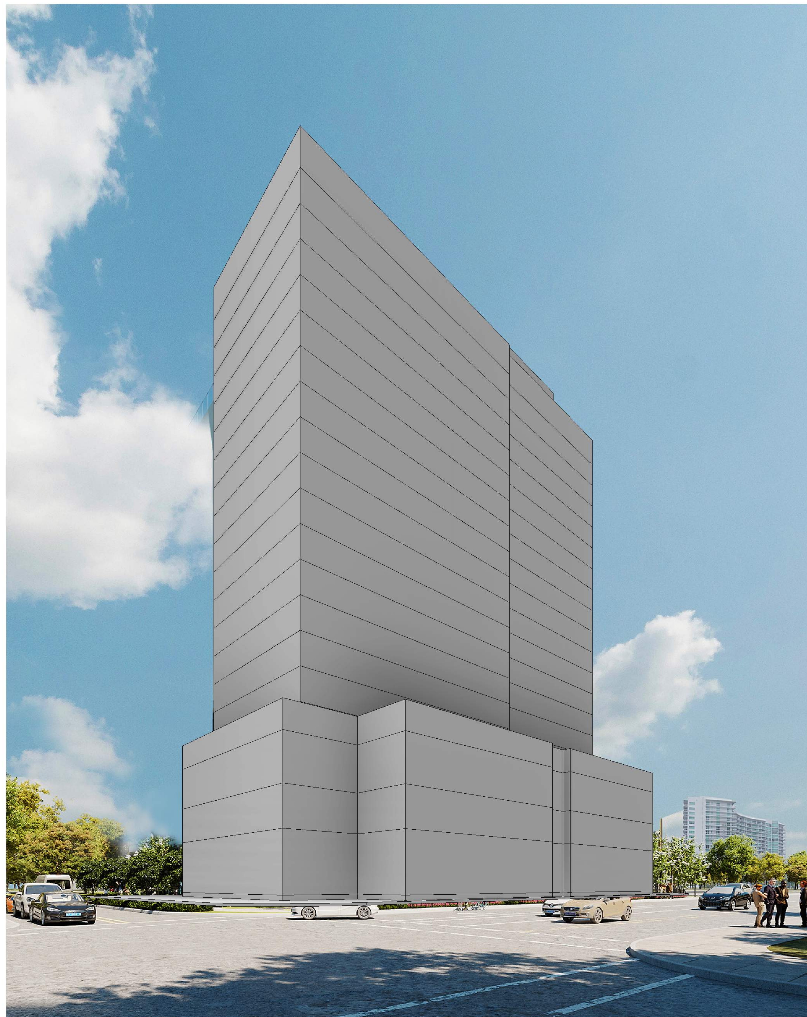
VIEW FROM SOUTH EAST CORNER - B2 BUILDING
