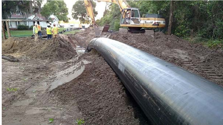
Our Task Order Manager Scott Richards' horizontal directional drill project under the Broward River in Jacksonville, Florida.
