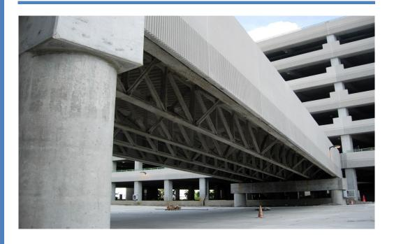
S&F Engineers, Inc. (SFE) provided structural design, construction administration support services and special inspection services under contract with Singer Architects for this bridge connecting the second floor of Hibiscus Garage with 3rd level of the Palm Garage. The new bridge made vehicular traffic between "short term parking" areas located at both garages possible.
