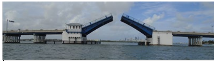
BROAD CAUSEWAY BRIDGE OVER ICCW
