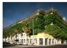
GREEN WALLS ON GARAGES
