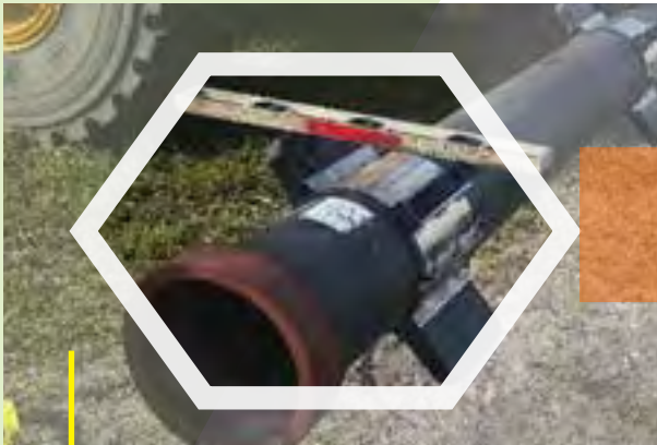
Pipe Spacers in Place for Casing Installation
