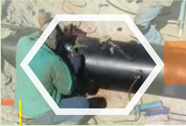
Welding Pipe Casing
