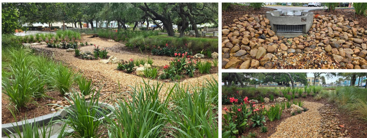
Figure 3-3. Green infrastructure like this smart rain garden in Veterans Memorial Park, City of Cape Canaveral is an example of Accommodation. Low impact development and green infrastructure in upstream locations reduce downstream flows by allowing more stormwater to infiltrate in place, thereby taking the pressure off the existing downstream stormwater infrastructure. (Photo credit: Zachary Eichholz, City of Cape Canaveral Chief Resilience Manager)
