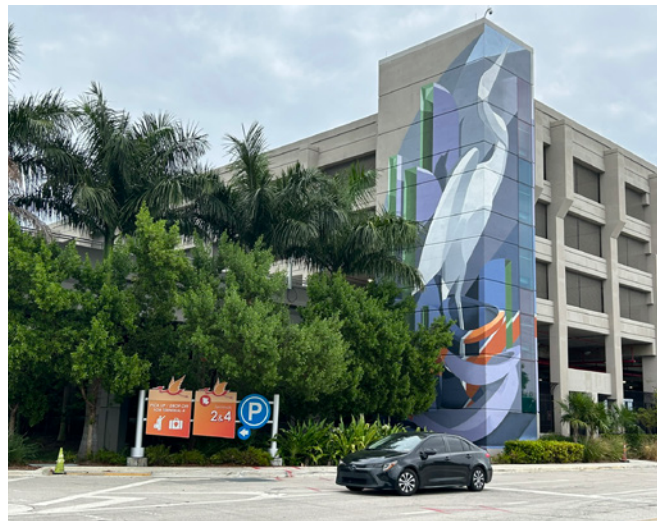
Port Everglades Terminal 2 & 4 Parking Garage Deck, Fort Lauderdale, Florida
