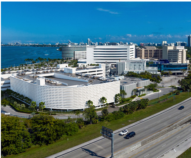
Mount Sinai Medical Center Parking Garage, Miami Beach, Florida
