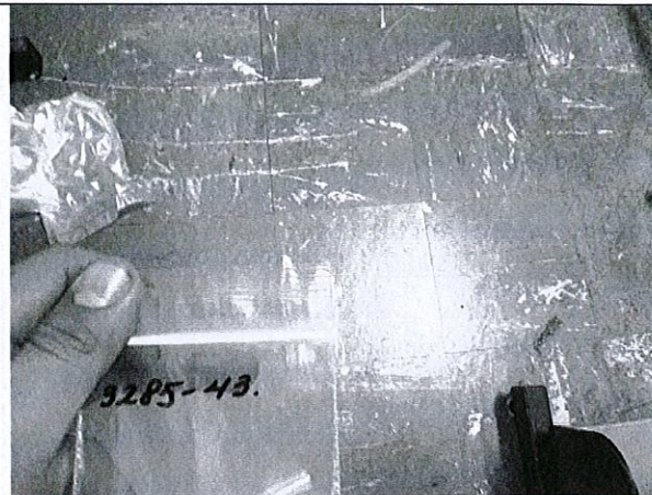
HA 18- Green 9" x 9" Vinyl Floor Tile Mastic is Asbestos Containing Material
