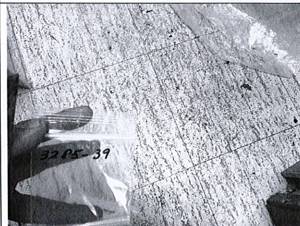
HA 16- White with Black Lines 12" x 12" Vinyl Floor Tile Asbestos Containing Material
