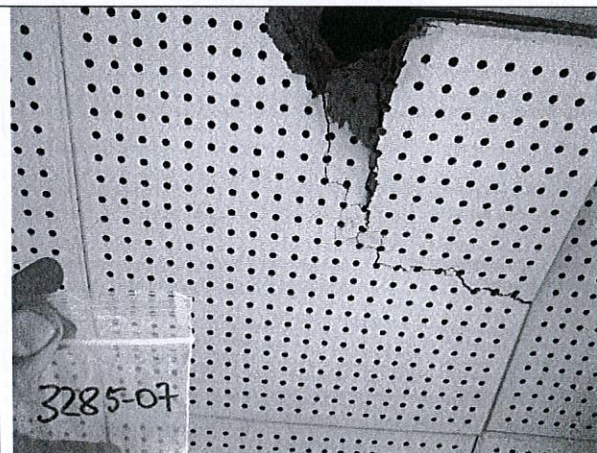
HA 3- White 12" x 12" Acoustic Ceiling Tile with Pinhole Pattern
