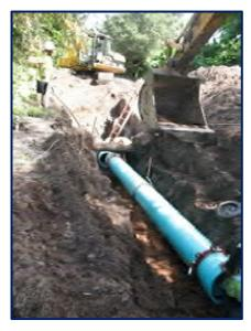
a nanofiltration concentrate pump station at the PGA WWTP. The blending station pumps nanofiltration concentrate from a lined holding pond at the PGA WWTP to the chlorine contact chamber at a controlled rate to optimize the conductivity/salinity of the blend water. A portion of this project was funded through an Alternative Water Supply Grant from the South Florida Water Management District.
