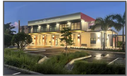
Tigner Community Center City of Deerfield Beach
