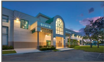
Civic Center Renovations City of Sunrise
