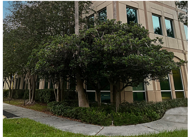
Broward County Property Appraisal Building, Fort Lauderdale, Florida
