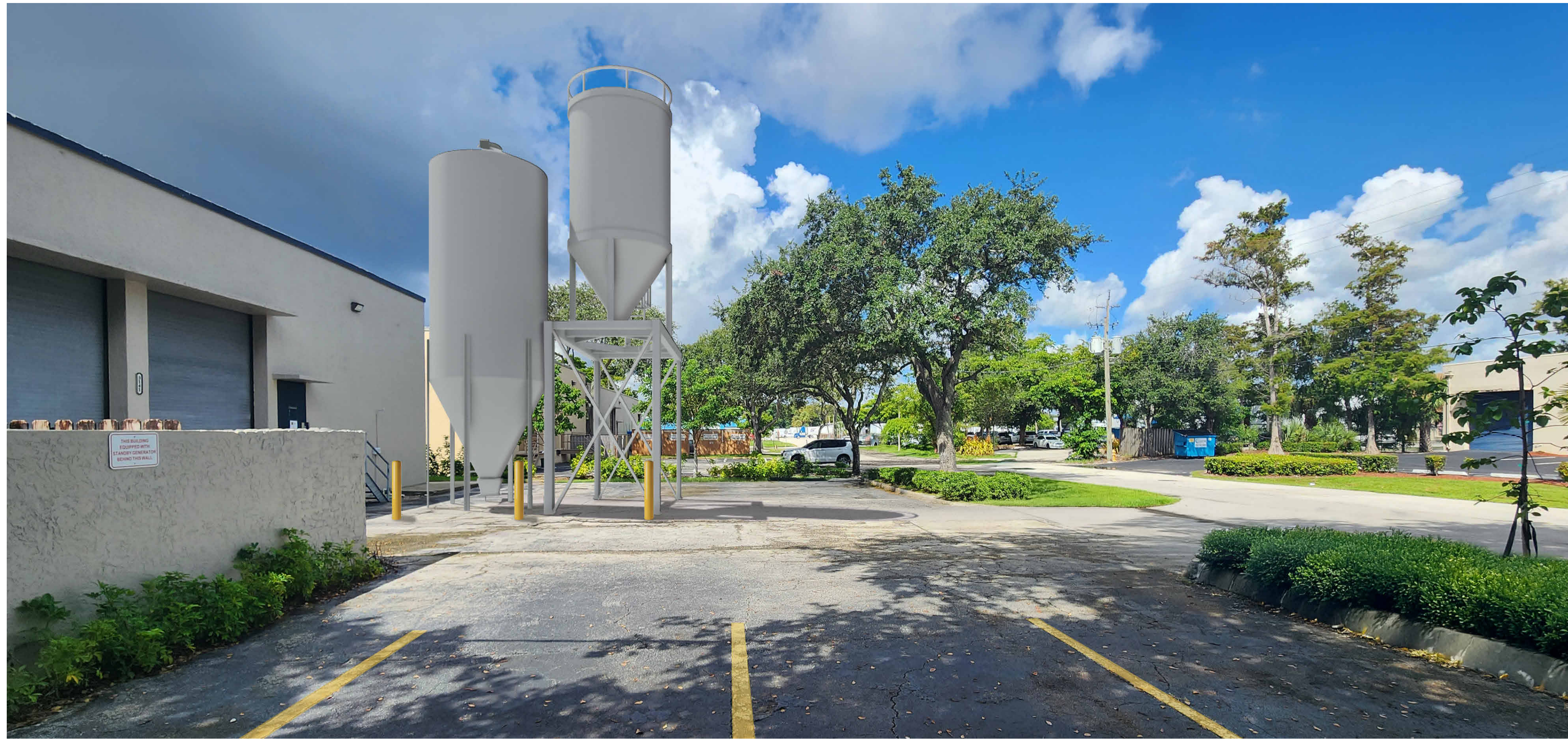
1 EYE LEVEL VIEW FROM PARKING SPOT AFTER PLACEMENT OF SILO SCALE: N.T.S.
