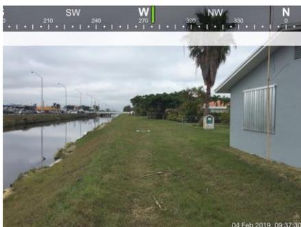
The C-4 Canal Bank Improvements - Palmetto Phase 2 Flood Protection Berm Project is located in Miami-Dade County, Florida and included the construction of approximately 2,545 linear feet of earthen berms on the north bank of the C-4 Canal between SW 87<sup>th</sup> Avenue and SW 82<sup>nd</sup> Avenue.
