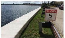
Cummins Cederberg was engaged to assess and rehabilitate an existing seawall for a waterfront condominium at the Intracoastal Waterway. A portion of the seawall was stabilizing the entrance road but had severely deteriorated, which could affect access to the property.
