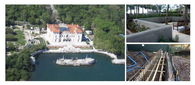
Cummins Cederberg was retained to determine potential storm surge impacts and design a wall to prevent damage to a restored historic garden.
