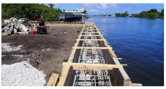
Cummins Cederberg was retained by the Colonial Club Condominium Association to perform an engineering inspection, which results led to the replacement of their 1,500-foot seawall with two return segments at the North and South corners of the wall. The property had experienced significant soil loss in several locations which was requiring persistent maintenance.
