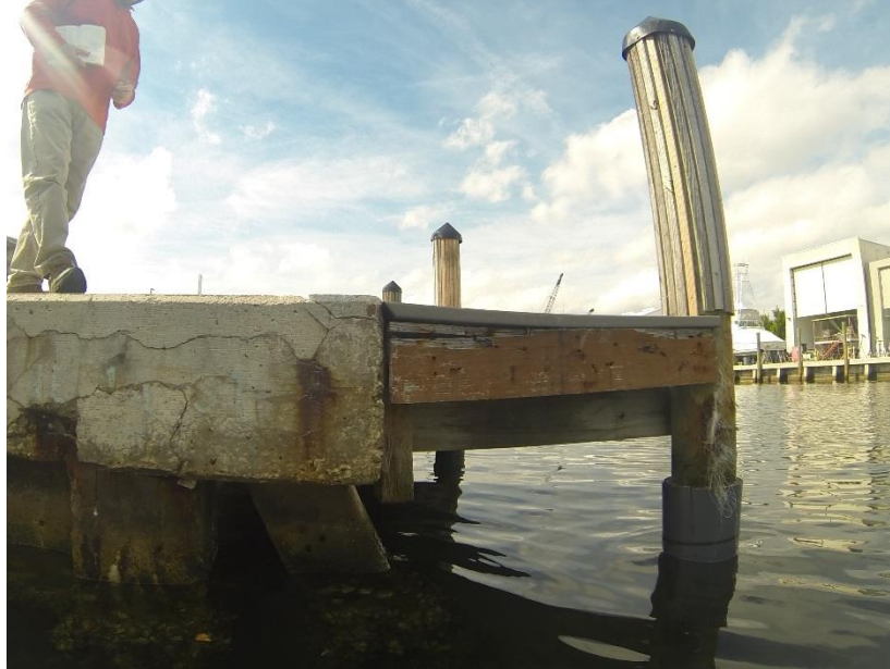
Plate C West View at East End along ICWW. Significant spalling, cracks and staining
