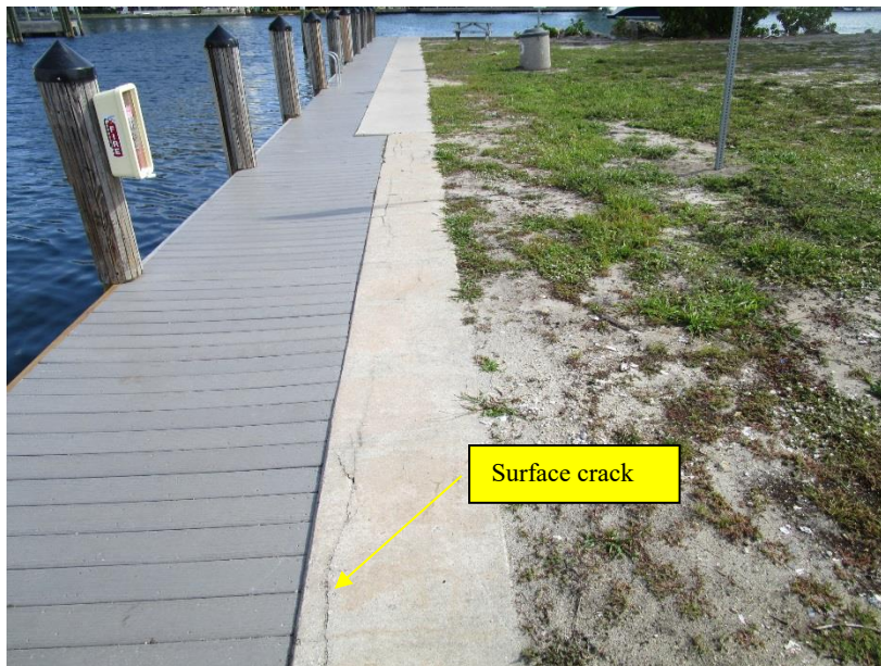
Plate J East view at transition from repaired bulkhead section to original bulkhead structure
