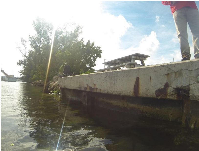
Plate B Southerly View at East End along ICWW. Significant spalling, cracks and staining
