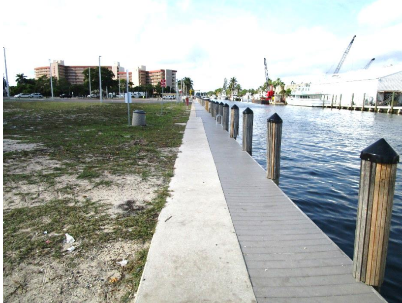
Plate E West View from East end of bulkhead
