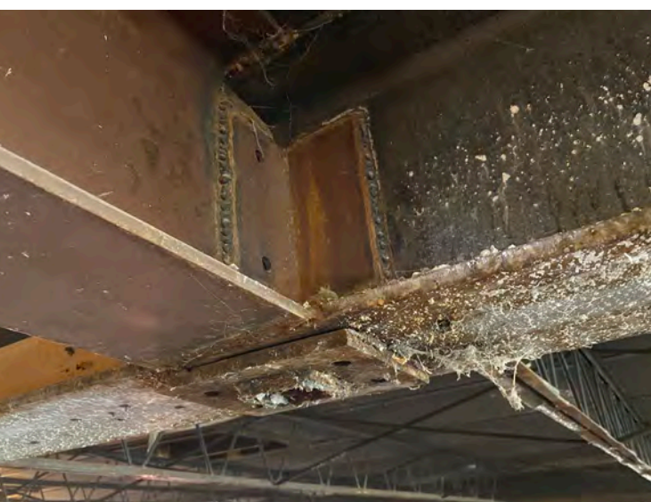
Discovery of a column which was removed during a prior remodel.
