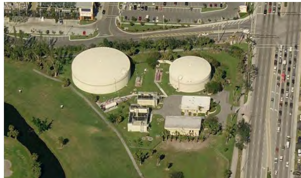
The City's Reclaimed Water Treatment Facility, one of the earliest in the region, provides reuse water through a progressive program.
