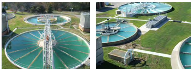
Lime softening basins operating in conjunction with Membrane Treatment at Olathe, KS, 37-mgd WTP.
