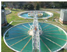
Lime softening basins operating in conjunction with Membrane Treatment at Olathe, KS, 37-mgd WTP.
