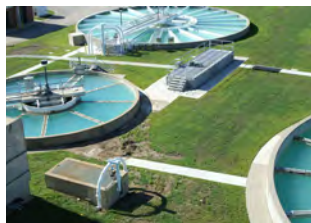
Lime softening basins operating in conjunction with Membrane Treatment at Olathe, KS, 37-mgd WTP.
