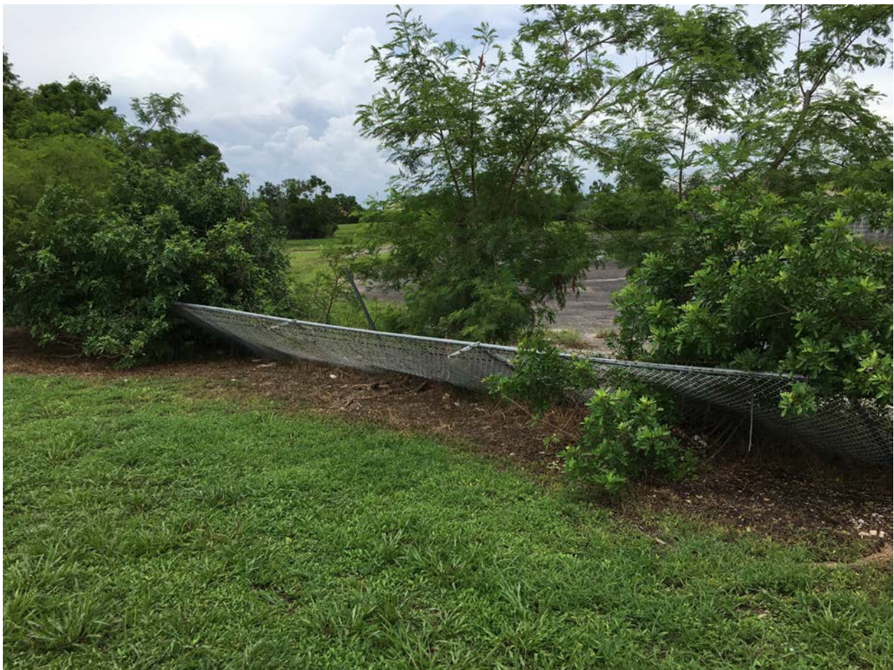
The West Boundary has sections of the chain link fence that are damaged and lying down.
