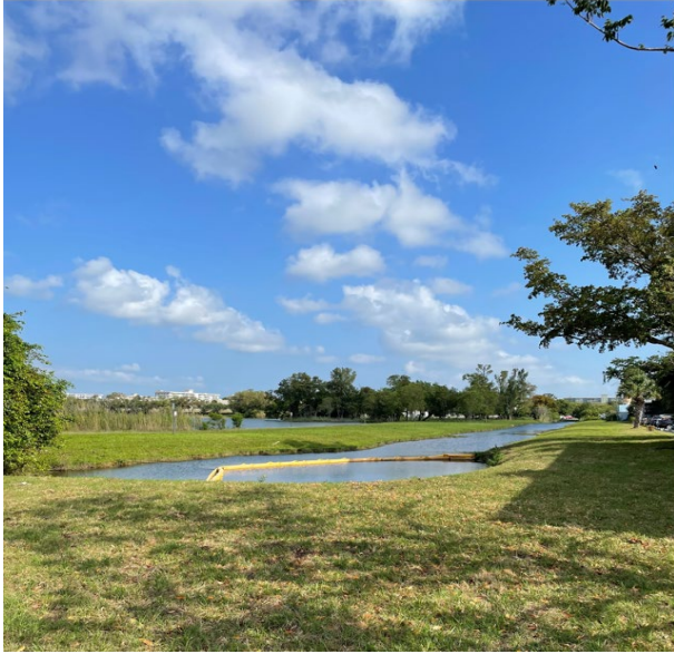
B-2 CANAL OUTFALL AT GATEWAY DRIVE
