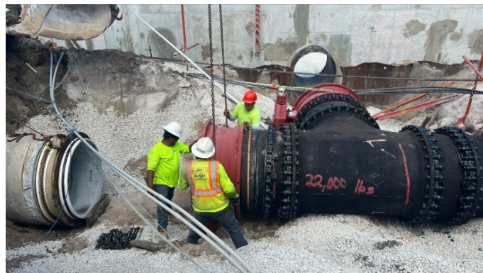
48-inch pipe tie-in
