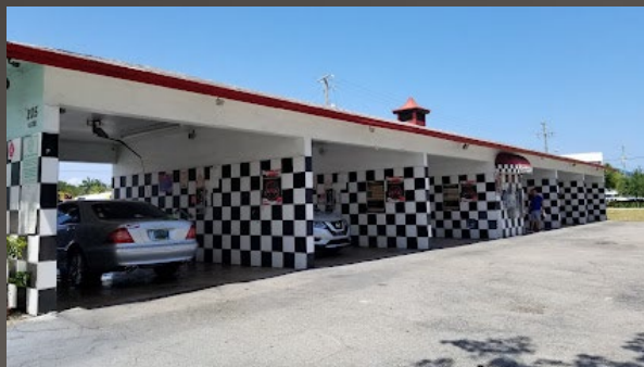
Car Wash – 205 E Atlantic Blvd
