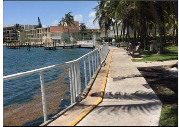
BULKHEAD & WALK ALONG WAHOO BAY
