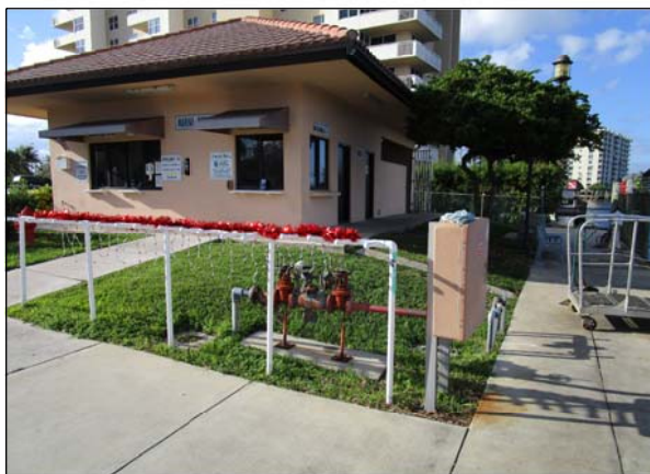
OFFICE / RESTROOM FACILITY
