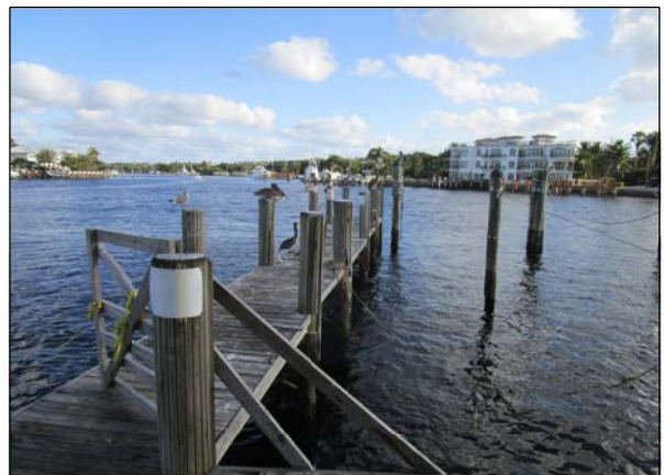
NORTH DOCK ALONG ICWW
