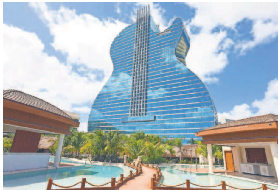
In addition to the 450-foot guitar hotel, the Hard Rock added the Oasis Tower, which houses 168 rooms and swim-up suites. SEMINOLE HARD ROCK HOTEL & CASINO
