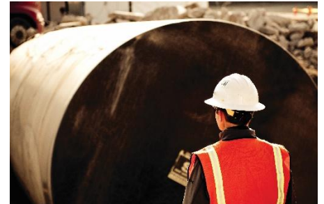
Terracon provides site investigation and closure services for underground storage tank removals.
