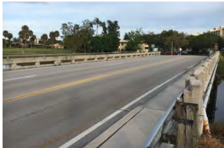
North Palm Aire Bridge
