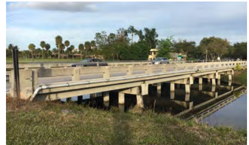
North Palm Aire Bridge
