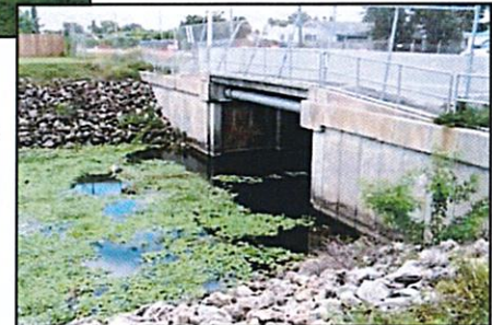
Lawrence Road Bridge over Boynton Canal
