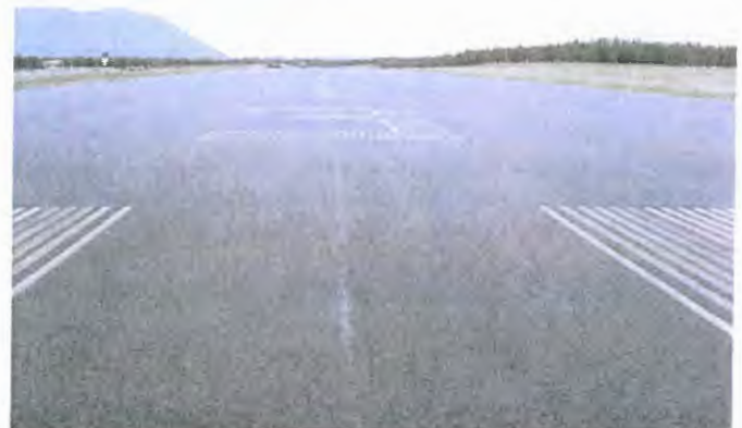
Reclamite application at this airport was completed in about one hour, and the stripping was left intact. The pavement's high void content—which allows fast water shedding in moist areas—eliminated the need for sanding after the application of Reclamite.
