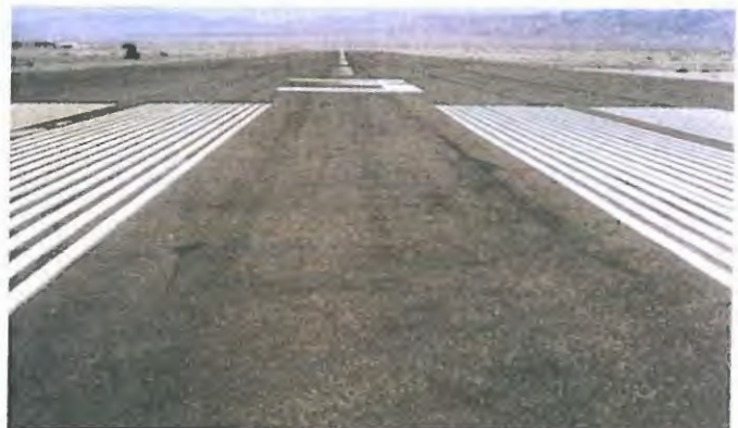
Reclamite preservative seal was applied to this ten-year-old asphaltic concrete pavement runway. Due to the dry, brittle pavement condition, total absorption of the Reclamite eliminated the need for sanding.
