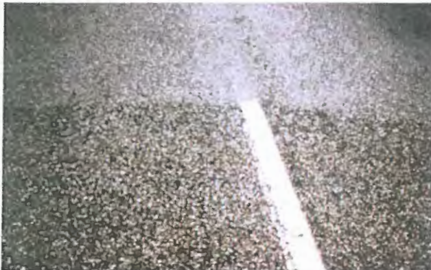
Reclamite was applied to the upper portion of this open-graded pavement; the lower portion was not treated. This photo, taken four years after application, shows severe loss of aggregate in the lower untreated area. The upper Reclamite-treated portion shows no surface loss or distress.
