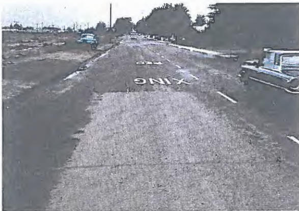
Reclamite was used as a construction seal on the dry areas of this pavement. Untreated areas are still wet from water penetrating the surface.
