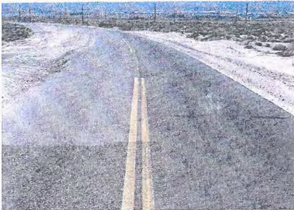
Reclamite was used as a construction seal. For comparison, the lower left area was not treated.
