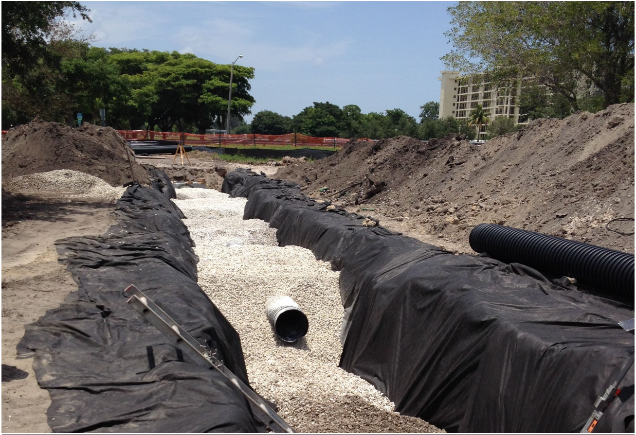
NEW DRAINAGE INSTALLATION
