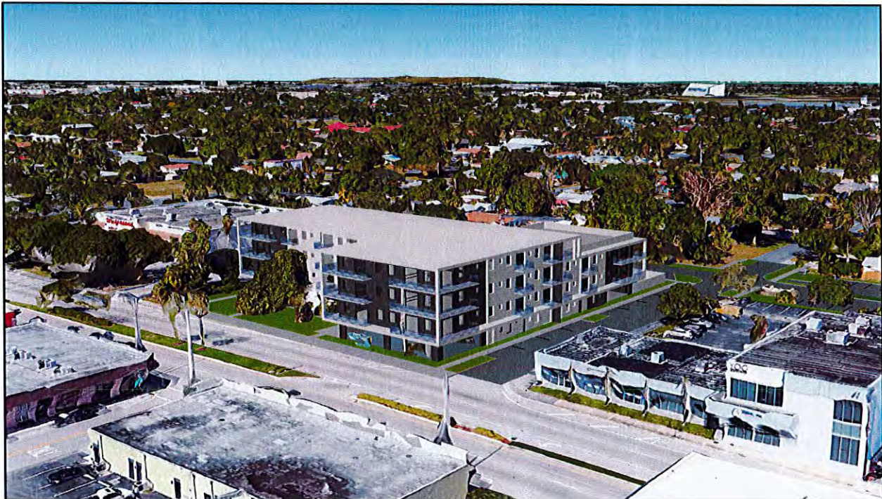
Figure 2 Birdseye view looking NW from E. Atlantic Avenue and NE 11th Avenue
