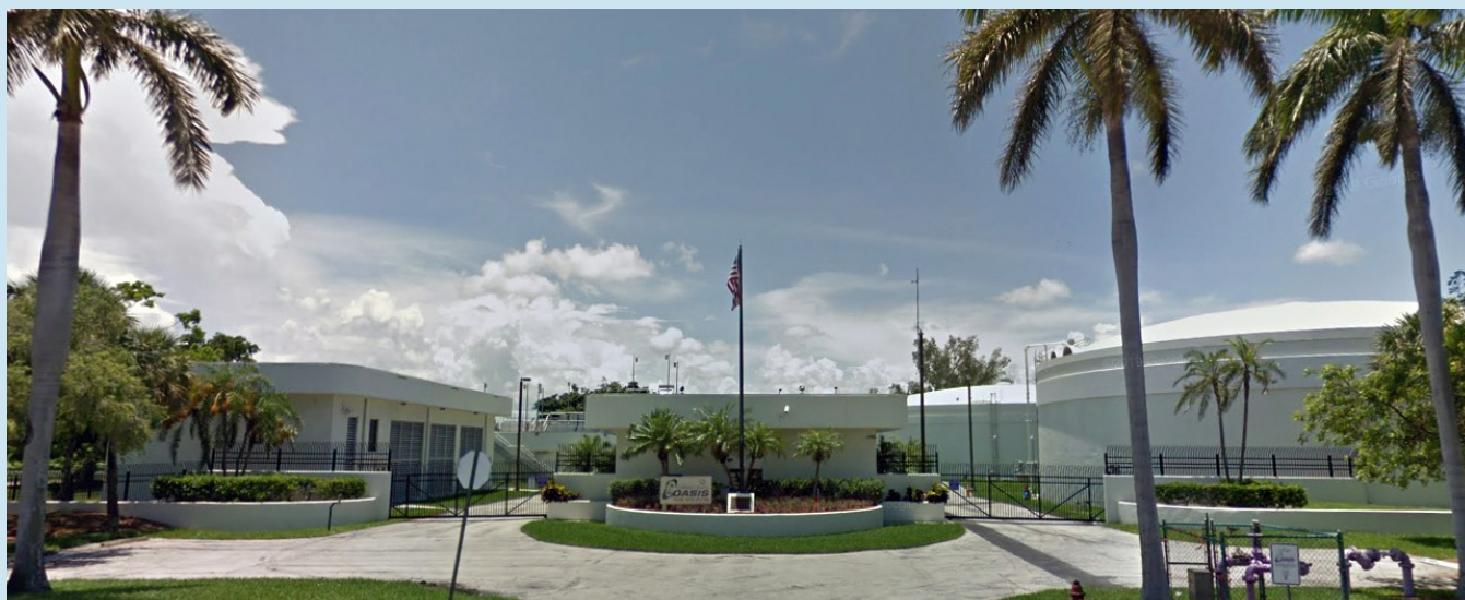
Oasis Reuse Treatment Plant
