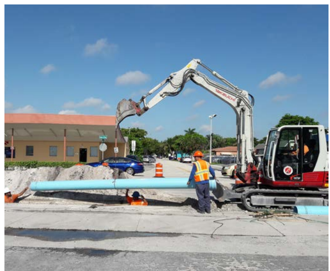
Water Main constructed in Broward County
