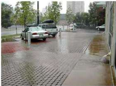
Figure 155.5102.C.2.b: Use of pervious materials in a parking lot.
